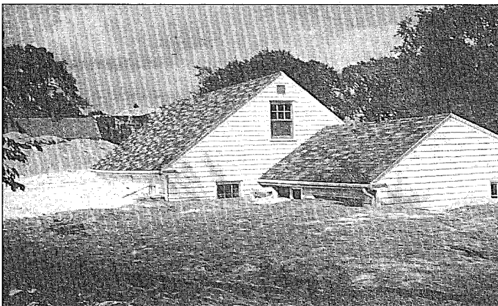
Figure 7. Large volumes of sediment can be deposited by floodwater during the course of an alluvial fan flood event.
